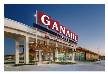
The new 18-acre yard in Torrance with 225,000 square feet of new buildings includes a retail store, will call storage and loading area, operations offices and two mezzanines. Using a composite design, the wood frame structure supports a concrete slab to provide for rooftop parking.
